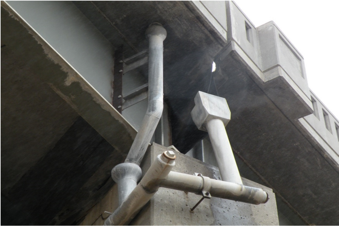
Figure 53 Drain Pipes and Overhang at Pier 8
