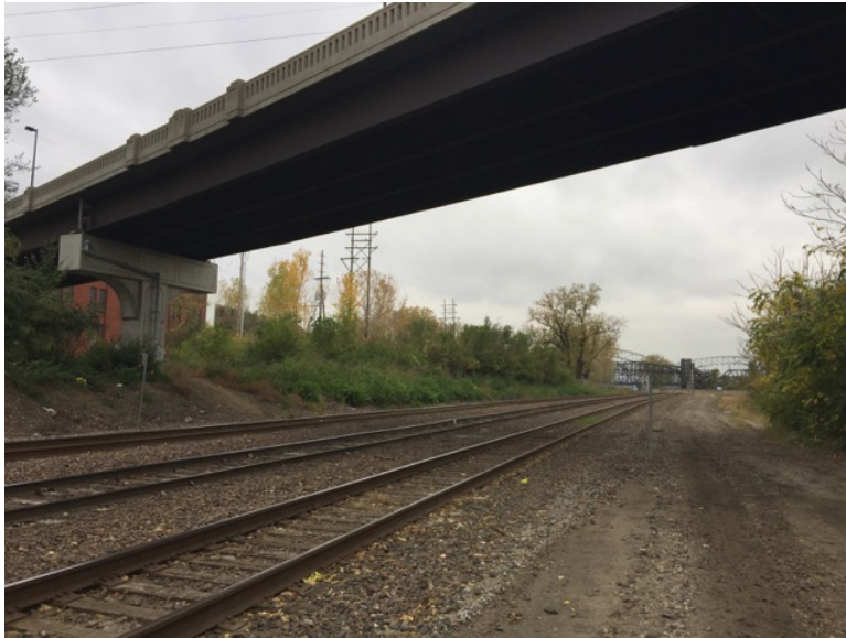
Figure 7 Railroad under the Grand Avenue Bridge
