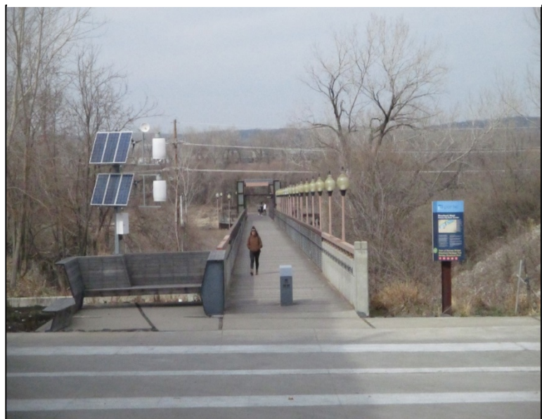
Figure 20 Town of Kansas Bicycle / Pedestrian Bridge
