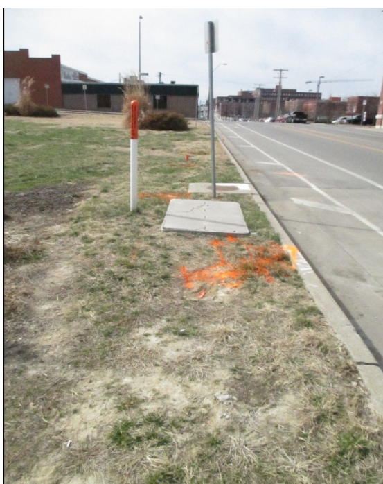
Figure 26 Missing Sidewalk on 3rd Street
