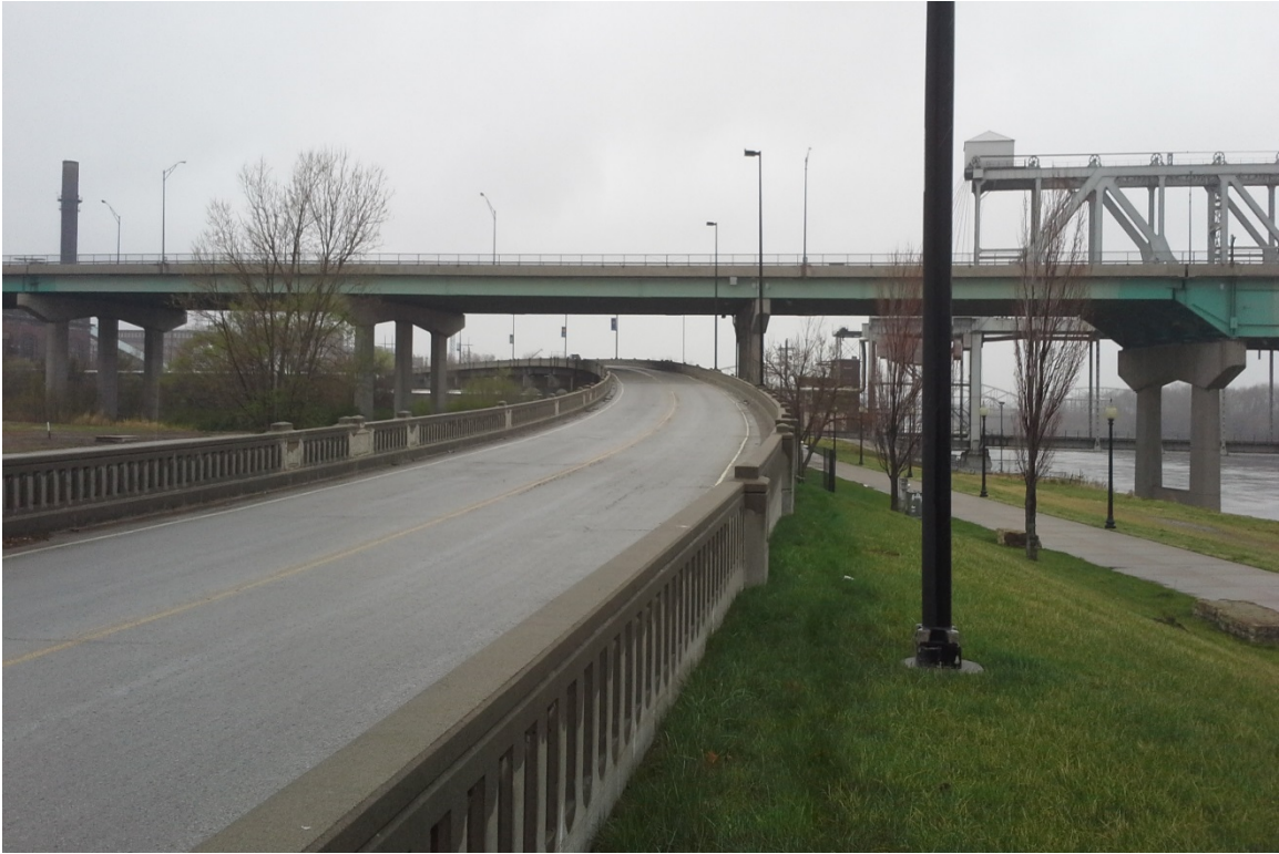
Figure 59 General View at North MSE Wall Segment
