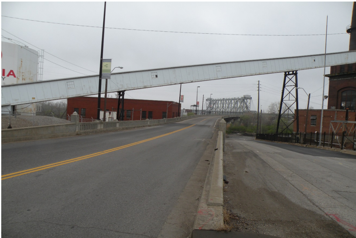
Figure 50 General View Looking North
