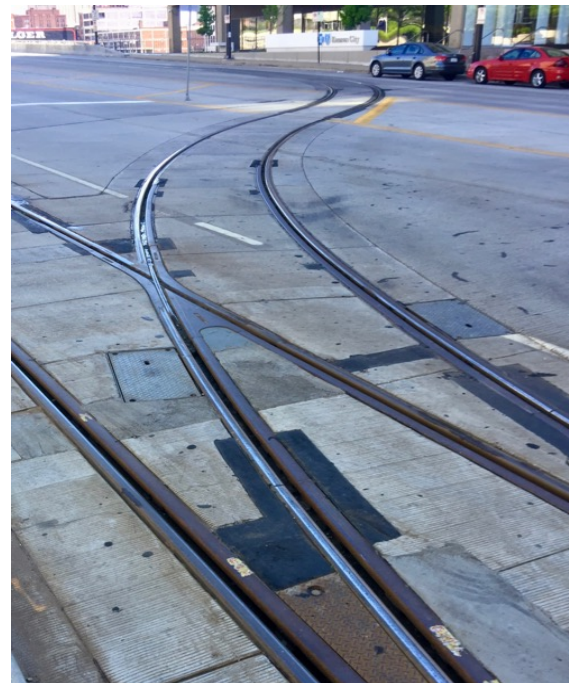
Figure 5 Frog and Turnout at Union Station
