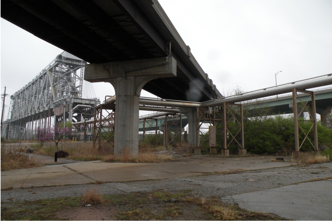
Figure 57 Piping under the Bridge
