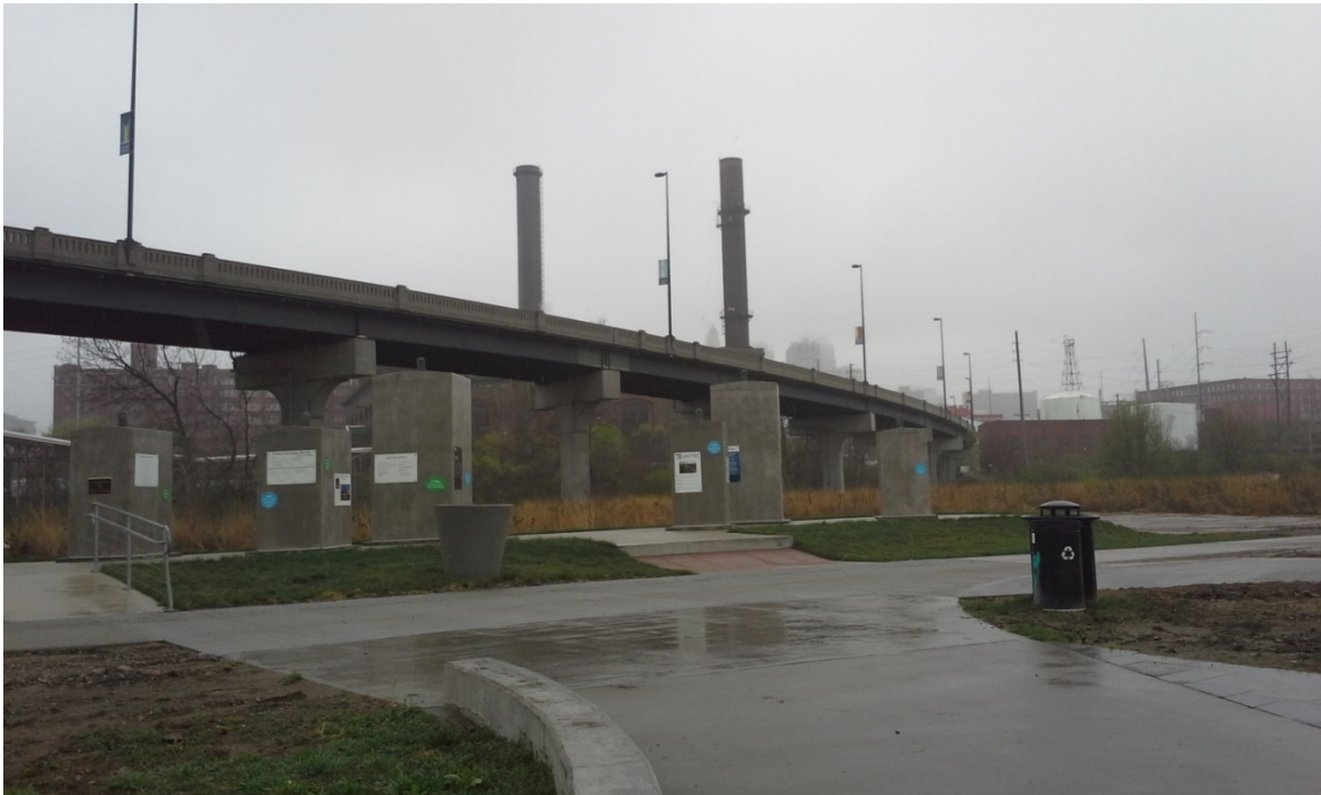
Figure 58 General View of North End of Bridge
