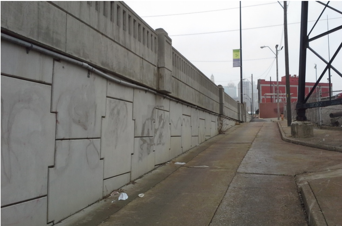
Figure 56 West MSE Wall near Abutment 1
