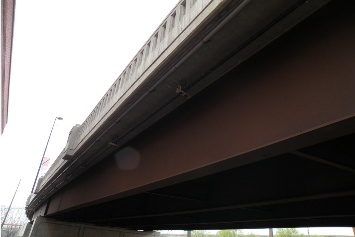
Figure 51 West Girder and Overhang with Utilities
